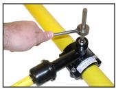
**14** Screw punch down until stop on drive key contacts the top of the saddle tee. The tap is now complete.
