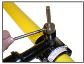
**15** To allow flow through service, back punch up until the top of the punch is flush with top of saddle. It is important that the punch does not protrude above the top of the saddle tee.
